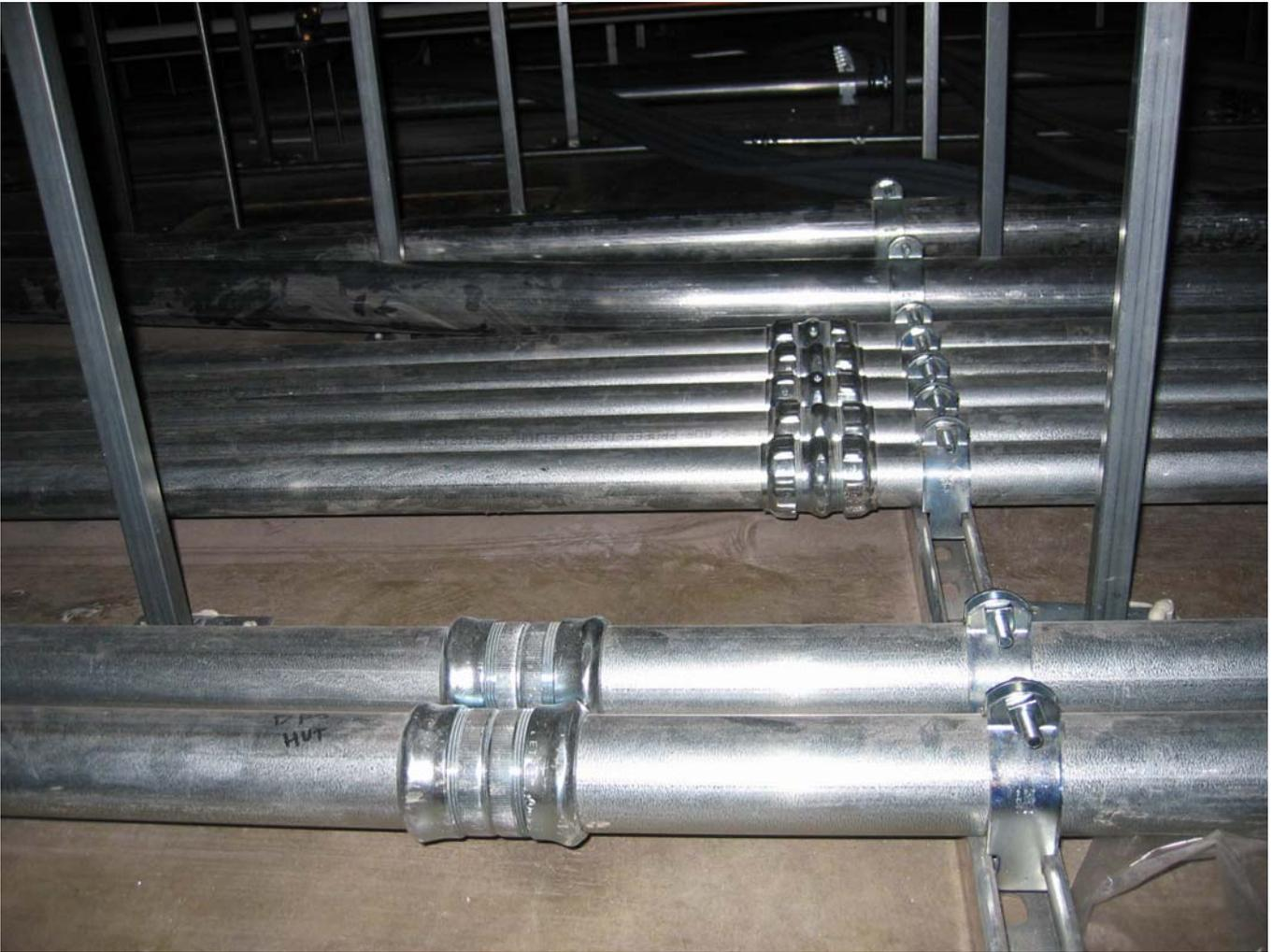
**FIGURE 3. Support of Components Off Floor**
