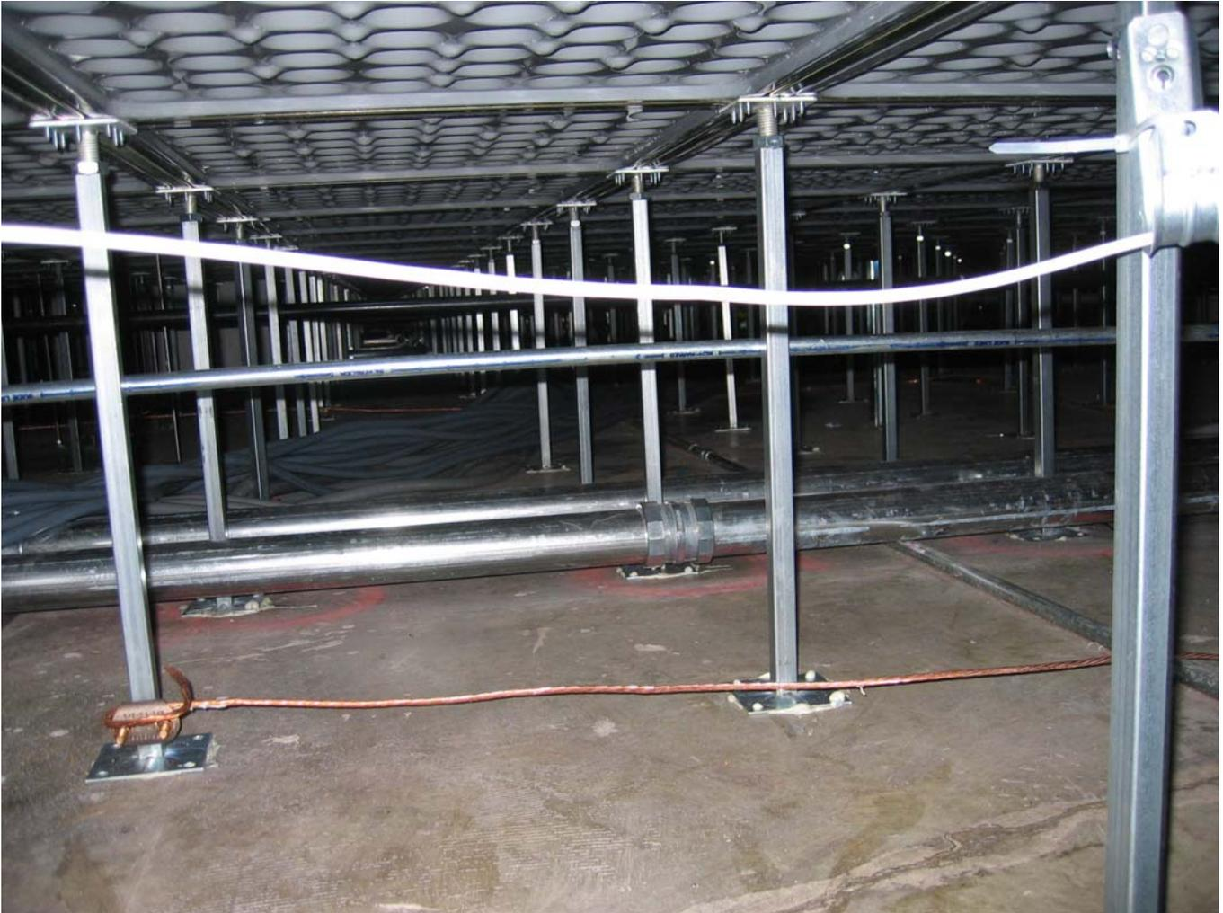
**ROUTE GROUNDING CONDUCTOR AT FLOOR LEVEL,
