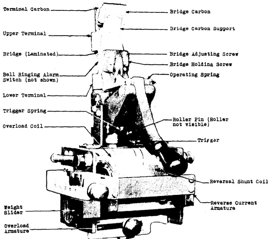
**Fig. 2 - Type EL Breaker - Overload and Reverse Current**
